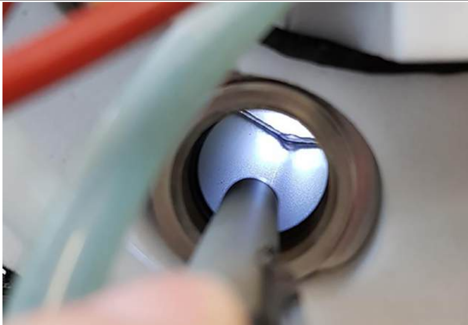
Inspection of the double jacket for deposits and corrosion
