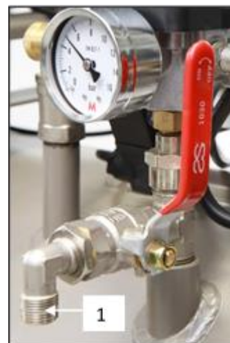
Fig. 8: Connecting to the compressed air outlet
