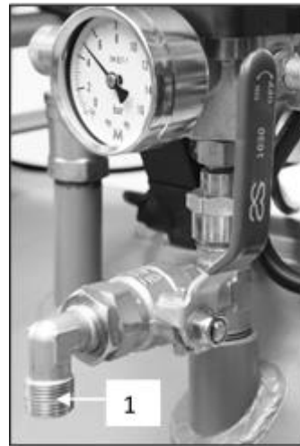
Fig. 8: Connecting to the compressed air outlet
